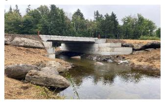
Precast box and arch sections are routinely used for streams spanning 4 ft to 22 ft. Available to come with or without a curb and guardrails are an available add-on. Rebar hoops are available for CIP curb attachment if our curb sizes don't meet your roads' requirements.
