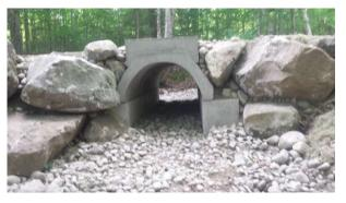
Depending on elevation of the stream design the CB blocks sit on abutment blocks with keyways so they nest together.
