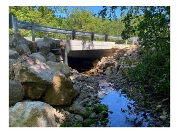
Our culverts fit on our Culvert Bearing (CB) blocks varying from 1' to 2' tall and 5' to 13' long with a 14" groove for the Arch/Box sections.
